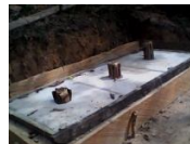
Toilet slabs in place with squothing holes marked
