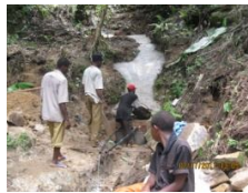
Constructing spring collection chamber
