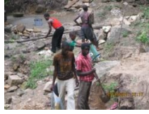
Constructing Egbea-chuk spring catchment
