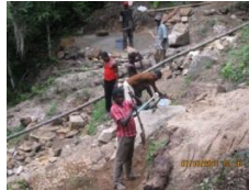
Laying bamboo pipe line to collection point
