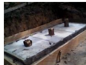
Toilet slabs in place with squothing holes marked
