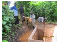
Casting toilet foundation
