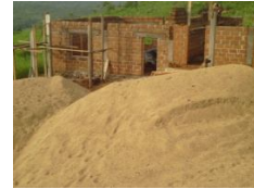
Sand on site
